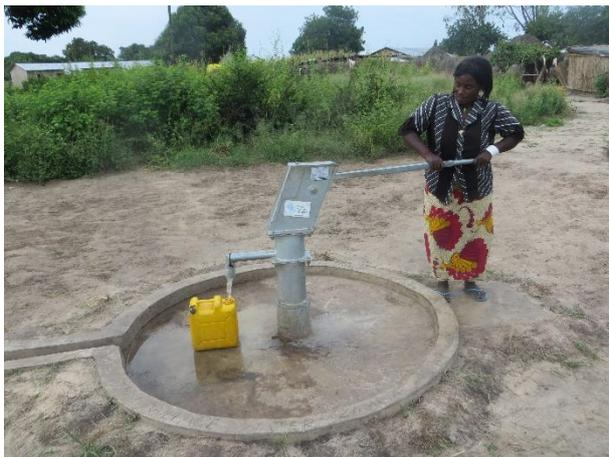
The community are now drinking safe water from a safe, protected well. The new well was manually drilled in January 2016 to a depth of 24 metres to future-proof it against climate change. It takes 3 strokes of the hand-pump to produce water and 45 strokes to fill an average 20 litre container. The water has been tested and is safe to drink.
