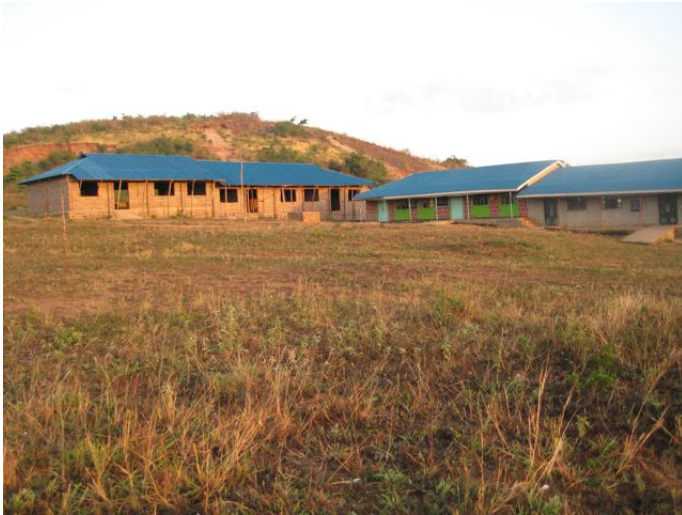
The school buildings – still under construction
