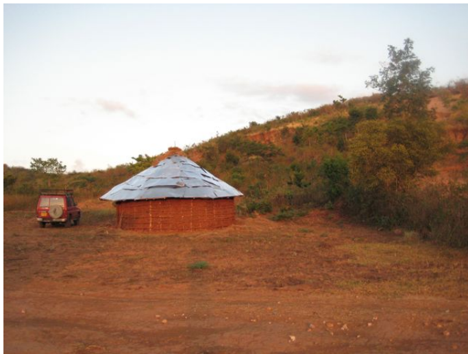
The Centre's office/our hotel! – still under construction
